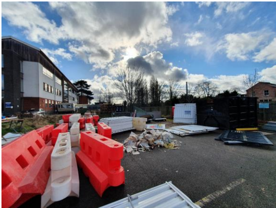
Facing south west (Y block to left)
