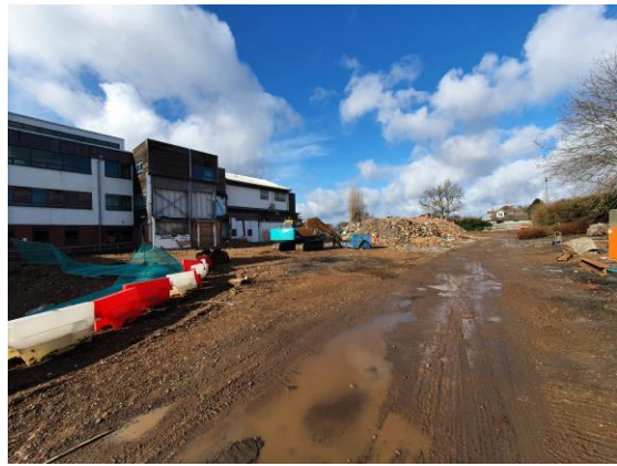
Facing north west (Y-block to left)
